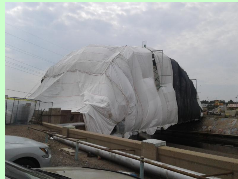
Truss bridge encapsulated
