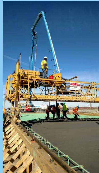
Pouring concrete on the southbound I-25 bridge over Indiana.
