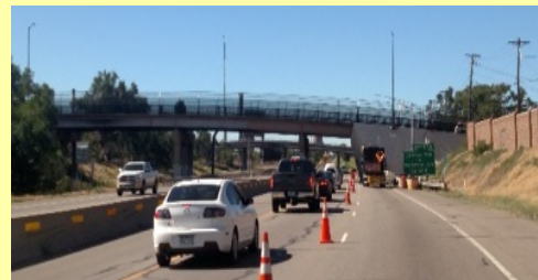
Traffic reduced to one lane on I-25
