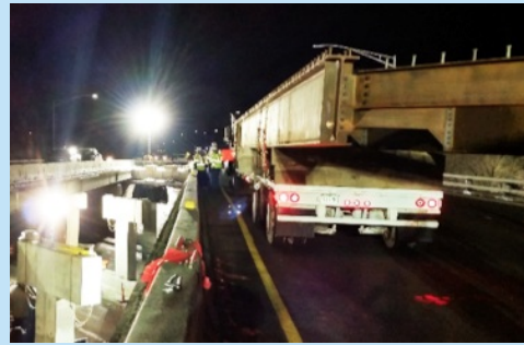
Steel I-girders at I-25 bridge over Indiana Avenue
