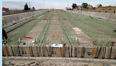
Box girders at I-25 over Gruma Drive
