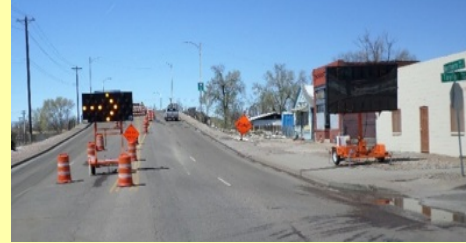
Rehabilitation work on Northern Avenue bridge over I-25
