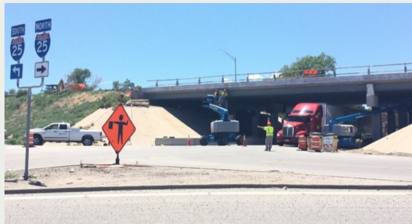
Work at I-25 bridge over Indiana Avenue
