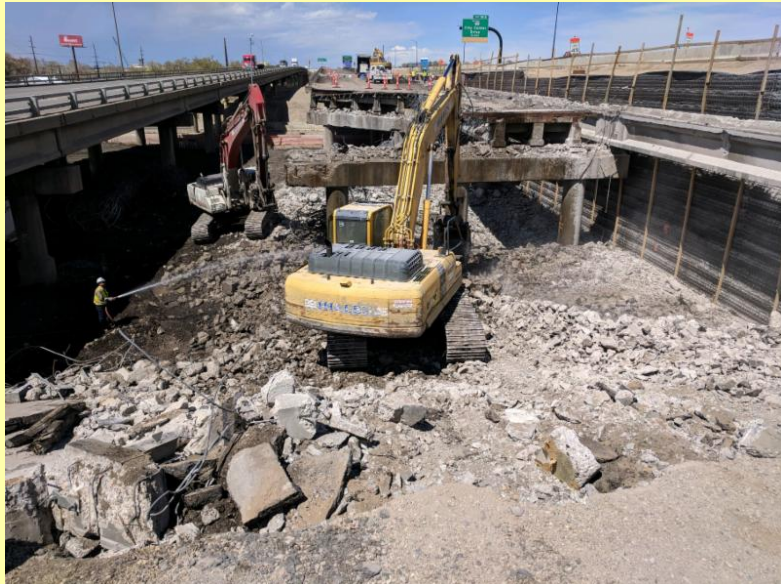
Demolition work in progress
