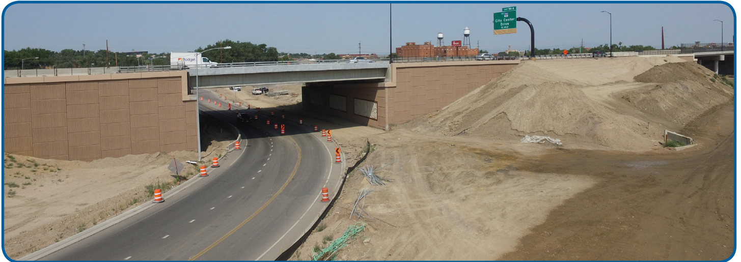
D Street bridge looking west
