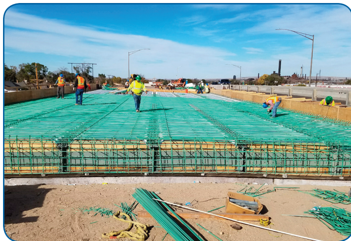
Deck construction on southbound I-25 over Indiana Avenue
