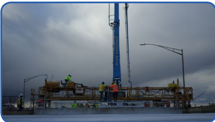
Paving northbound bridge at Indiana Avenue
