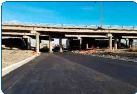
Newly paved D Street extension below I-25
