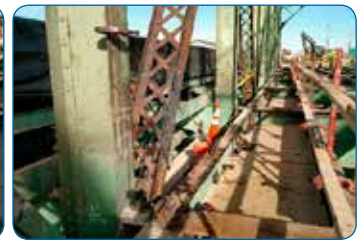
US 50 C Green Truss Bridge heat straightening before and after
