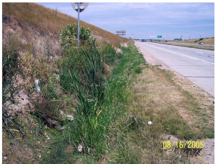
Typical Roadside Ditch
