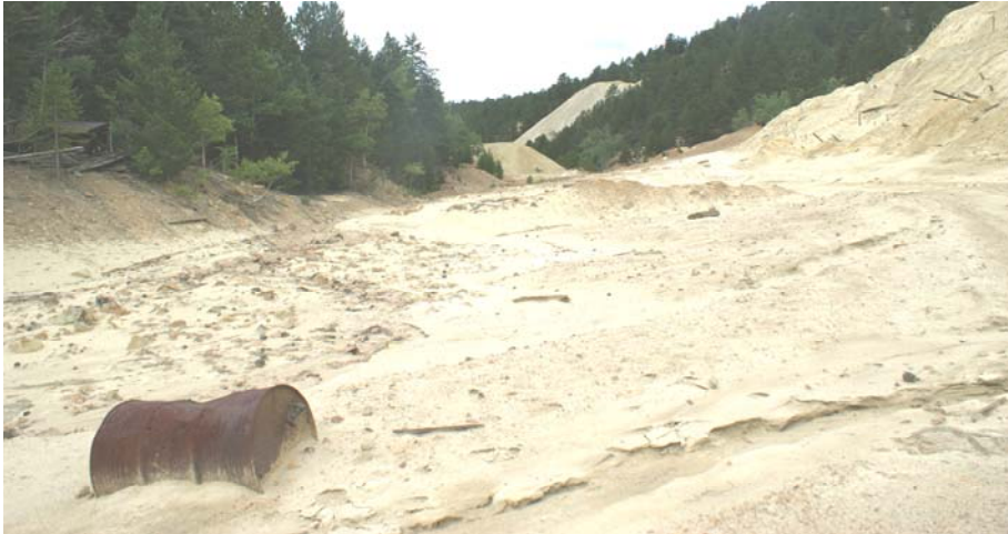
The sediment-choked channel of Russell Gulch illustrates the need to manage the flow of contaminated runoff as it travels downstream to the North Fork of Clear Creek.
