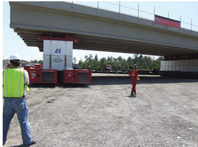
*Example of Self-Propelled Modular Transporters (SPMT)*
