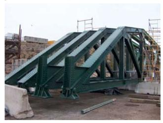
To preserve the history and character of the steel trusses, the Town of Estes Park will incorporate the trusses into their pedestrian trail system. Currently, the truss are being restored and being painted dark green (see photo above).
