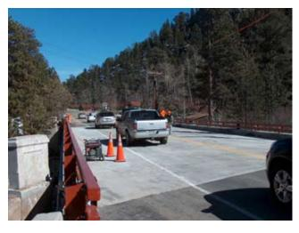
Since the completion of the new bridges, crews have been working on various construction activities including storm drain pipe installation, reconstruction of approximately 300 feet of roadway at each bridge approach in order to match the elevation of the new bridges, installation of new guardrail, and staining the new bridge concrete. Much of this work just got underway as crews had to wait for warmer temperatures to return and the ground to unthaw.
