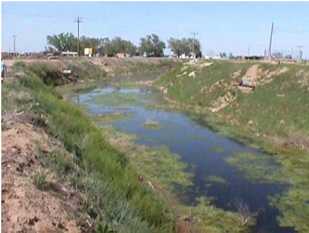
LAMAR CANAL, VIEWED FROM NORTH BANK TOWARD EAST
