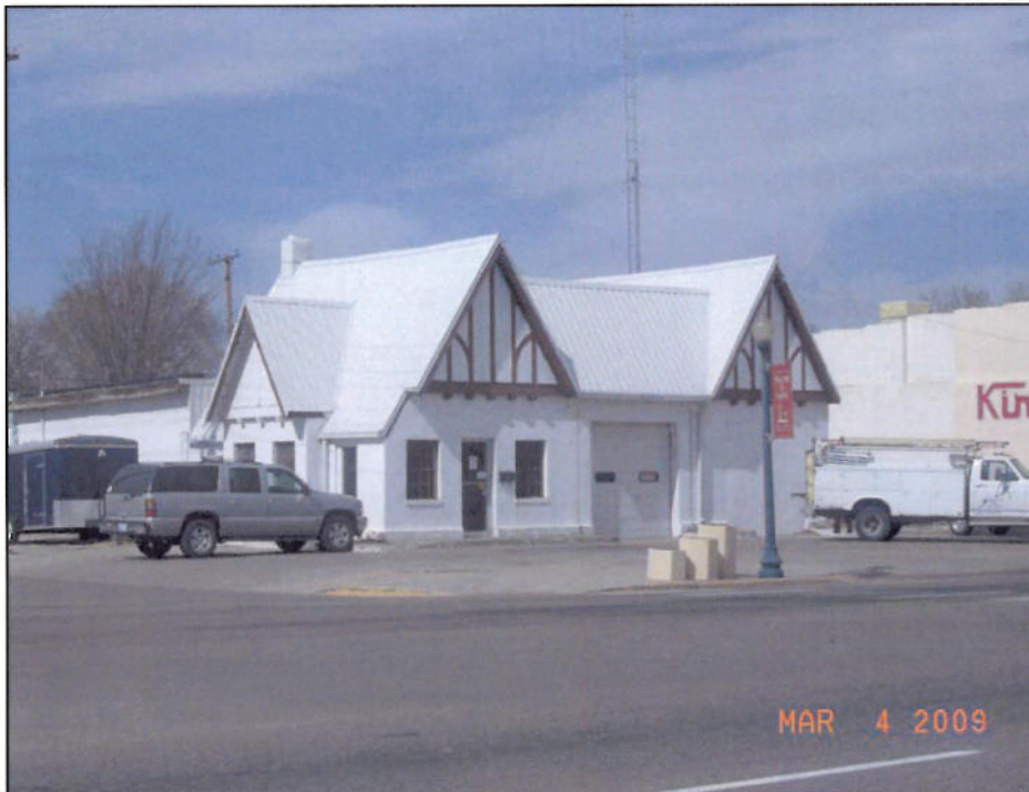
12 201 N. Main Street Gas station 2009-3, 76 1928
