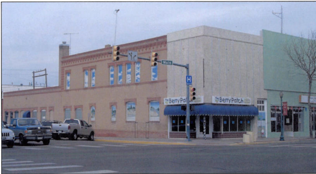
Image Date: March 4, 2009 Image By: Jennifer Wahlers, CDOT Figure 6-9. Looking NW at corner of Olive and Main Street
