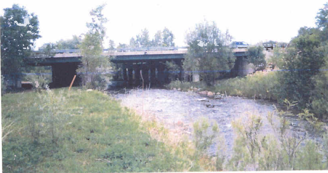
14. South Boulder Creek Bridge, looking downstream
