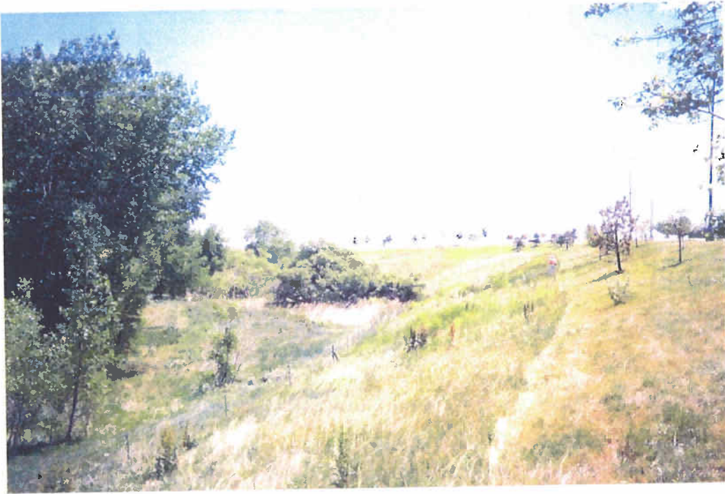
5. Rock Creek culvert, from west (Interlocken) side
