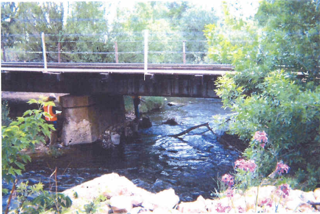
11. Railroad bridge over Boulder Creek
