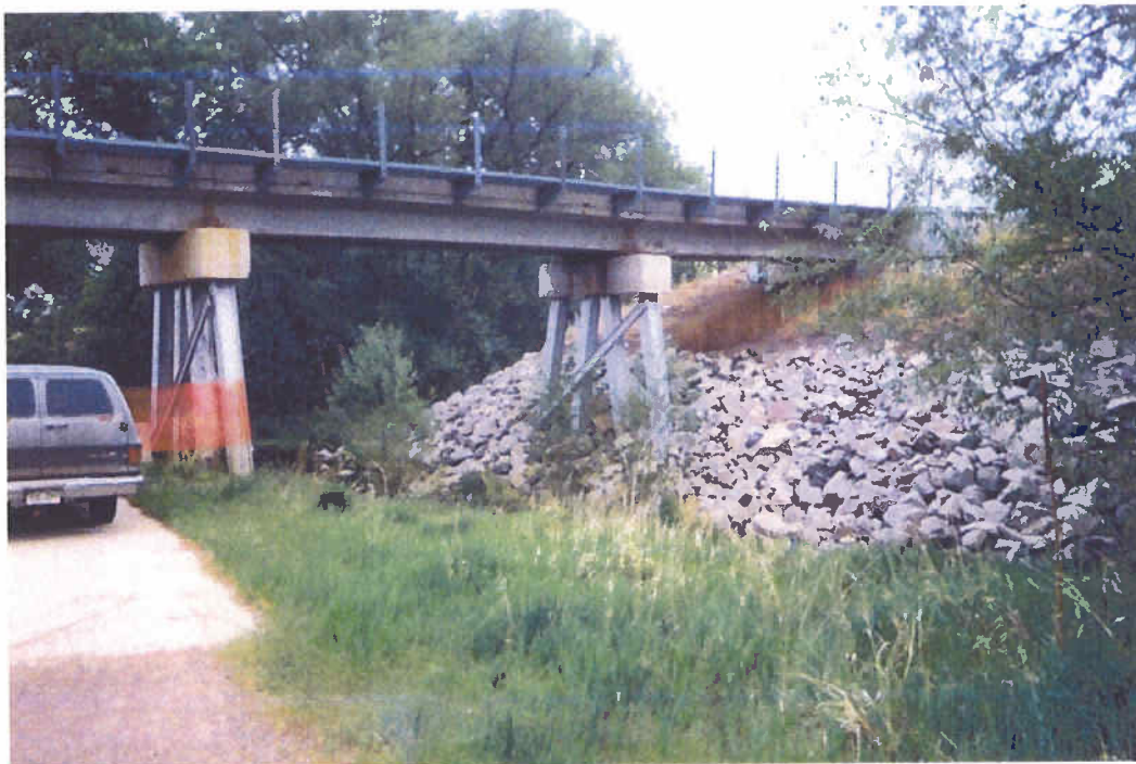
9. BNSF railroad bridge over Coal Creek
