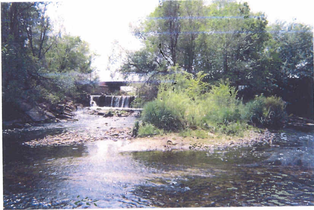
3. Clear Creek, looking upstream to railroad bridge and dam
