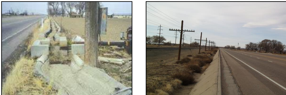
Figure 2-4. Examples of Inadequate Clear Zones on US 50
