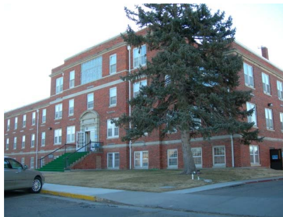
Figure 4-51. Arkansas Valley Regional Medical Center—La Junta
