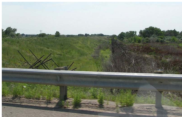
Figure 4-29. Arkansas River Levee—Las Animas
