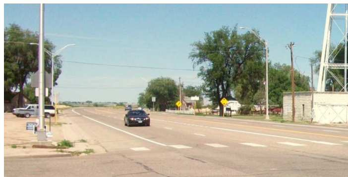
Four-Lane Segment of U.S. 50 with a Turn Lane (Swink)
