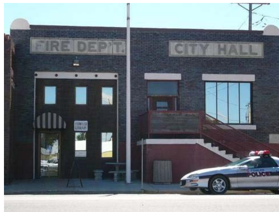
Figure 4-50. City Hall, Fire Department and Library—Fowler
