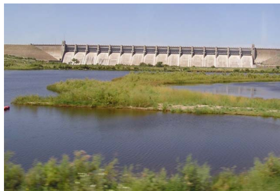
Figure 4-34. John Martin Reservoir—Bent County
