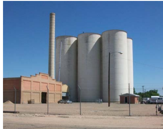
Figure 4-9. Agricultural Product Storage Facility—Rocky Ford
