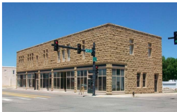
Figure 4-30. Avoided Historic Resource (I.O.O.F. Hall Lodge No. 11)—Las Animas
