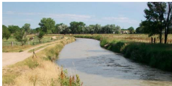
Figure 4-60. Catlin Canal (View from U.S. 50)—Otero County
