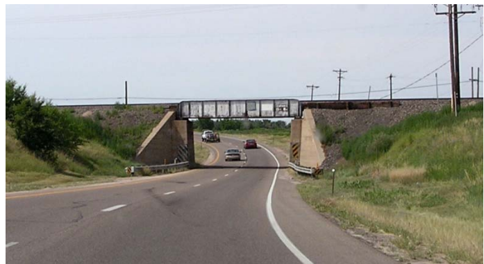
Figure 4-28. BNSF Railway Crossing of U.S. 50—La Junta
