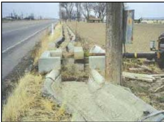
Figure 4-81. Examples of Inadequate Clear Zones on U.S. 50
