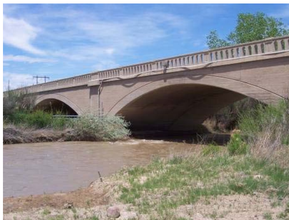
Figure 4-27. U.S. 50 Bridge over the Huerfano River (5PE.302)—Pueblo County
