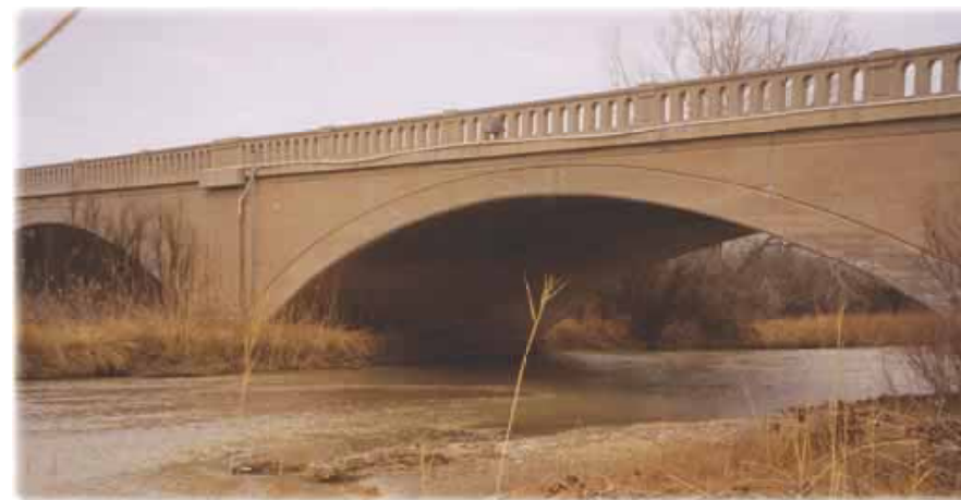
Historic Bridge over the Huerfano River
