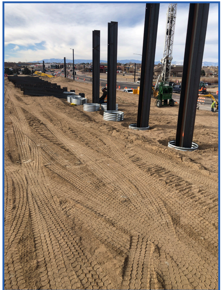
Work continues on the construction of bridge abutments.
