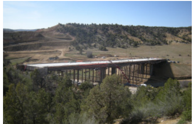
US 160 bridge construction in Grandview
