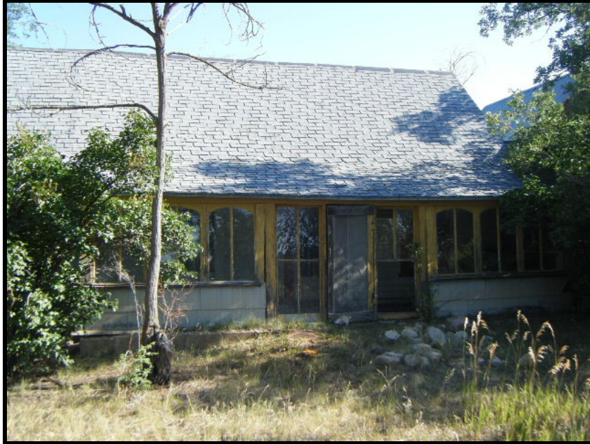
Figure 10. Residence (Structure 3) on site 5LP9306, photograph looking northeast at south elevation.
