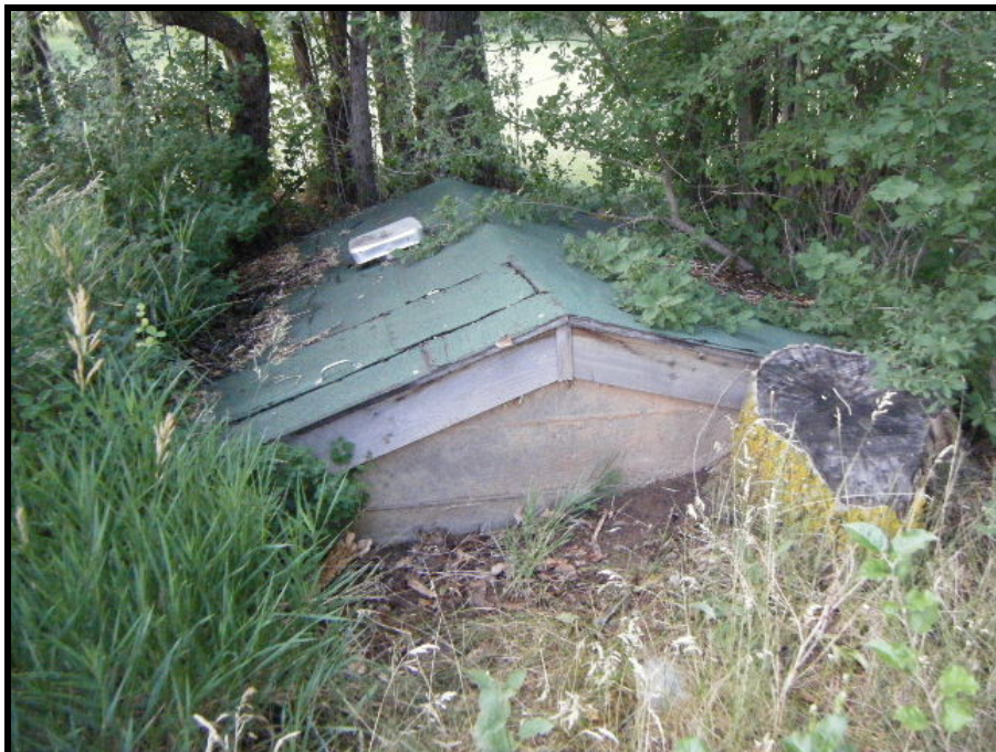
Figure 15. Pump house (Feature 1) on the Clark Property (5LP9310), photograph looking south.
