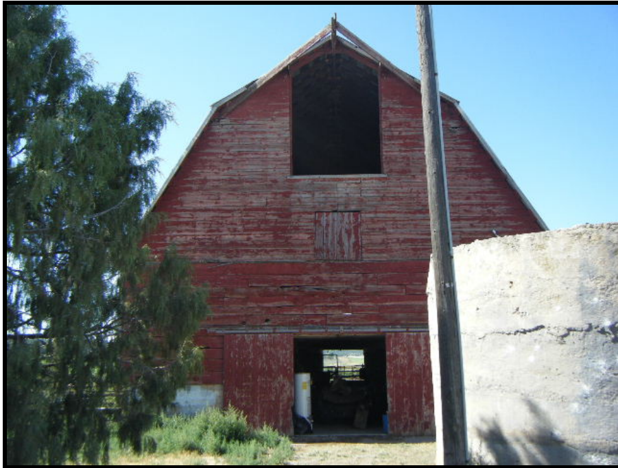
Figure 11. Photograph showing the barn (Structure 1) on site 5LP9307, photograph looking south showing north elevation of the barn.
