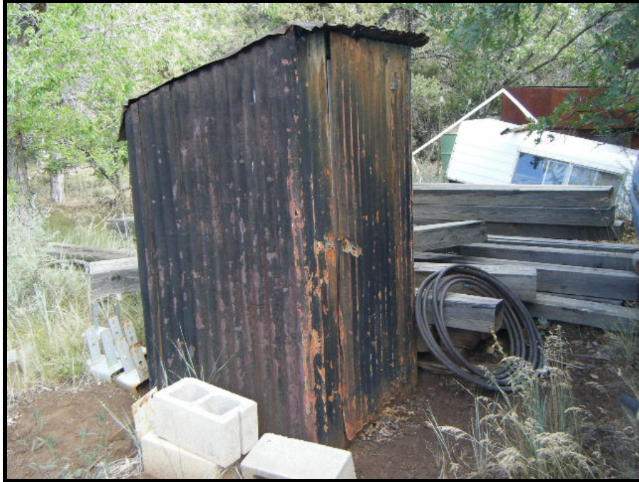
Figure 14. Outbuilding (Structure 2) on the Clark Property (5LP9310), photograph looking northwest.
