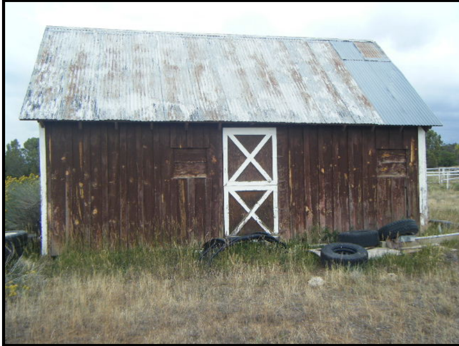
Figure 13. Photograph showing the saddle shed (Structure 4) on site 5LP9307, photograph looking north at south elevation.
