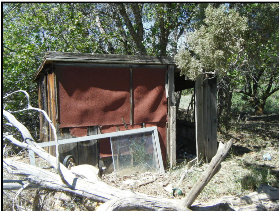
Figure 3. Photograph of Structure 8 (chicken coop) on site 5LP9307, looking southwest.
