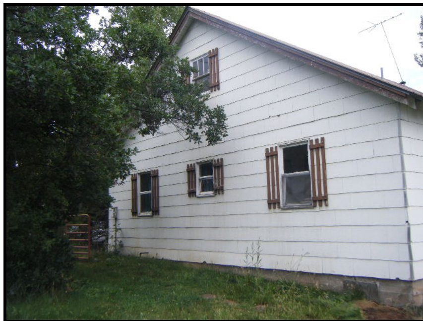
Figure 10. Residence (Structure 1) on the Clark Property (5LP9310), photograph looking southwest at the east elevation of the original house.
