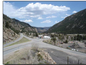
CDOT MAINTENANCE FACILITY AT I-70/US 40 INTERCHANGE
