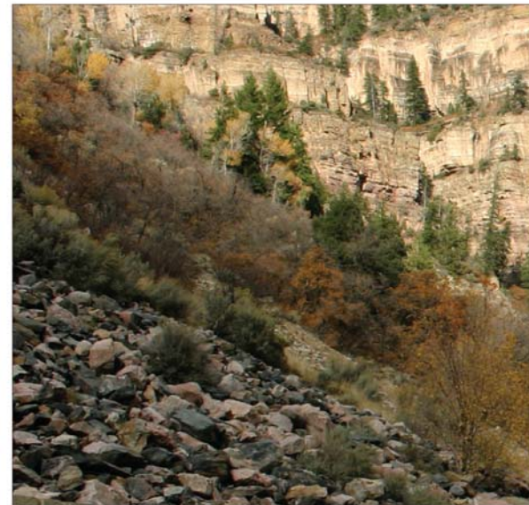
B | Boulders and talus rock used in conjunction with native planting will stabilize and restore steep slopes to a more natural condition.
