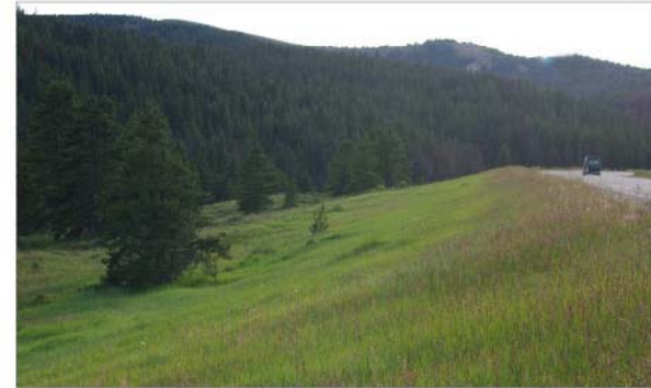
A | Rounding the top and toe of the slope blends embankments into the existing landscape and facilitates revegetation of constructed slopes.
