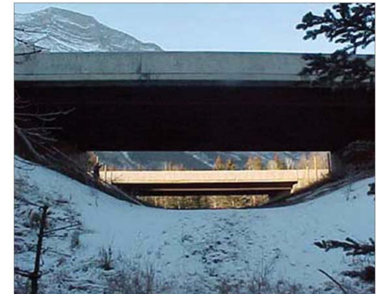
D | Underpasses that utilize open-span bridges offer greater visibility for wildlife than box culverts or enclosed crossings.
