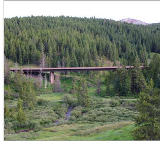
A | Roadway and bridge design should consider naturally occurring landforms and wildlife movement patterns.
