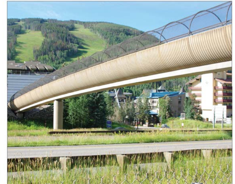
C | Pedestrian bridge crossings reconnect the community when bisected.
