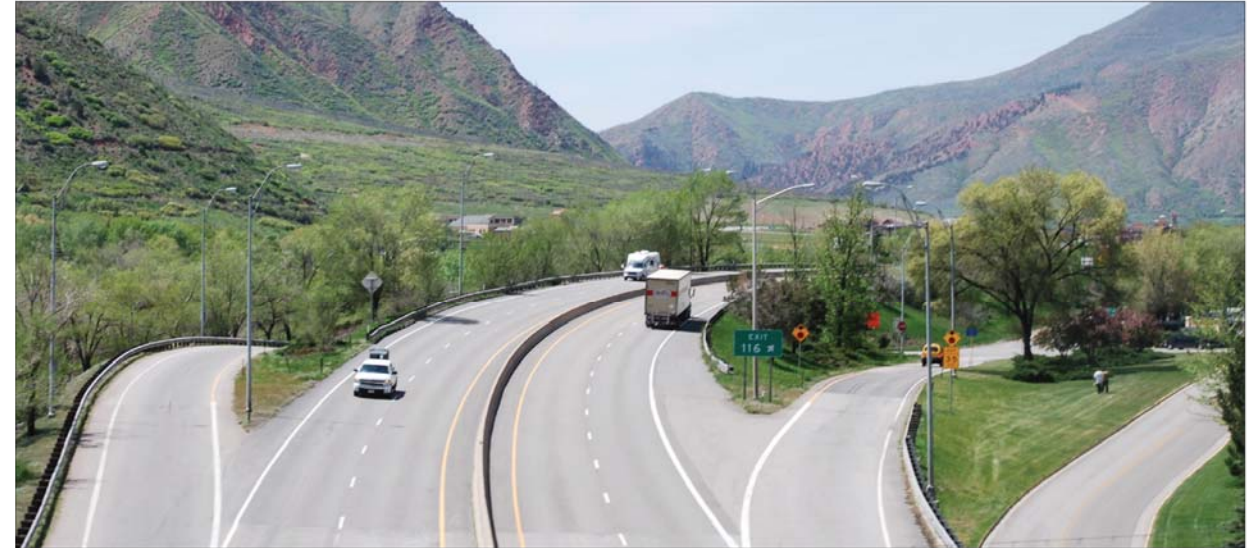
A | Interchanges should exhibit a compact design and include dense landscaping in open areas to create a transition from the transportation corridor to the community environment.
