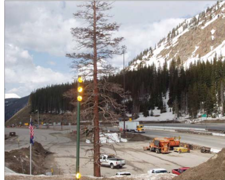
A | The approach to the Eisenhower Johnson Memorial Tunnel presents a cluttered and confusing mix of construction and maintenance uses to the traveler.
