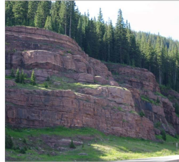
A | Rock cuts should include naturalized benches with planting pockets to mimic the surrounding landscape.
