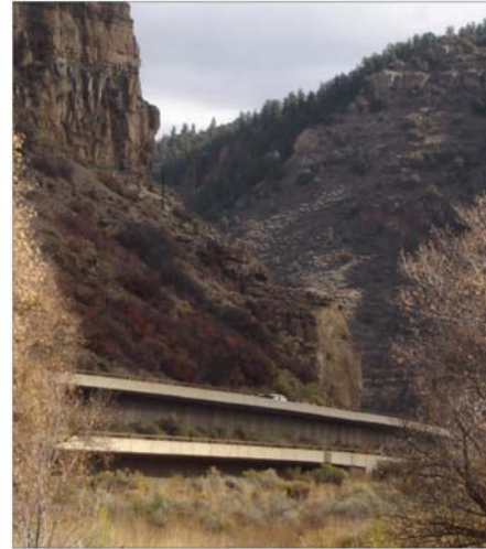
A | Using a split elevation for the travel lanes will adapt the corridor to the steep slopes found in this segment.
