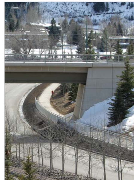
B | Community circulation must be considered at the onset of interchange design to ensure the creation of comfortable pedestrian spaces.
