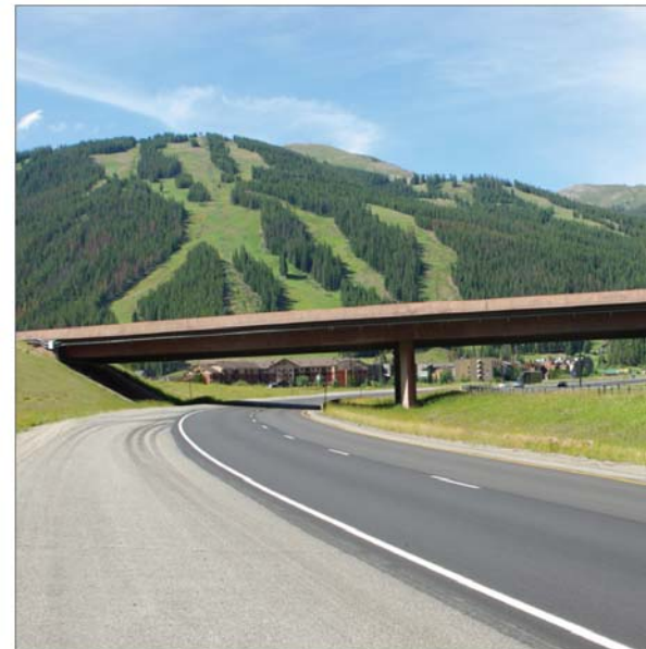
B | The bridge at Copper Mountain presents an aesthetic character with color, shadow, and box girder construction.
