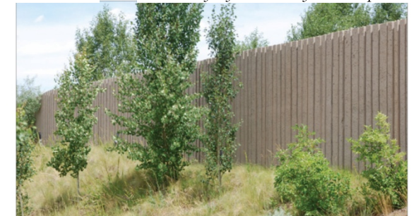
D | When sound walls are required, utilize berming, landscape, texture, and limited wall height.
