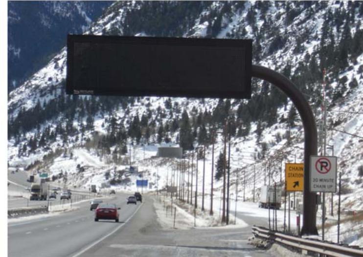
A | Single-arm monotube systems should be used.
