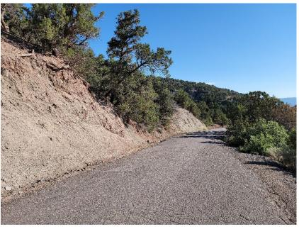
Photo 2. Steep slopes with weakly cemented surficial soils
