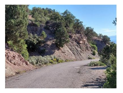
Photo 4. Rock outcrop and weakly cemented surficial soils
