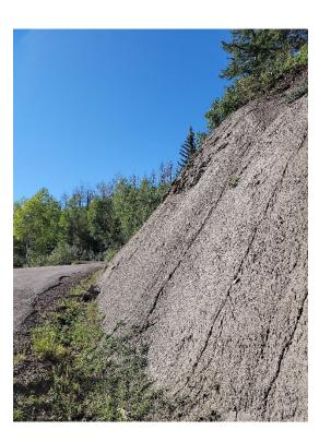
Photo 6. Closer look at steep slope surficial conditions. Note the erosion from surface runoff.
