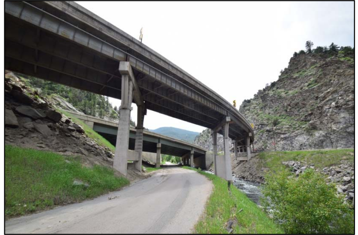
Existing I-70 bridges spanning the bike path, Clear Creek & the I-70 westbound on-ramp.
