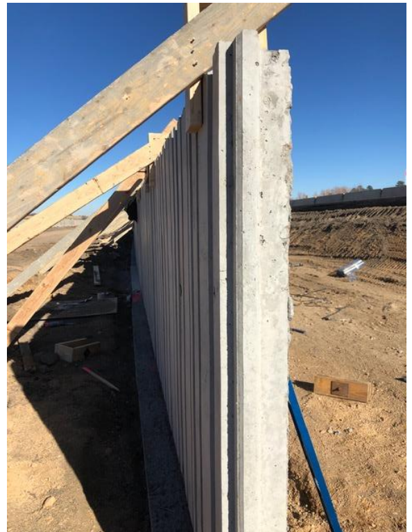
These walls are foundational to the new roadway.
