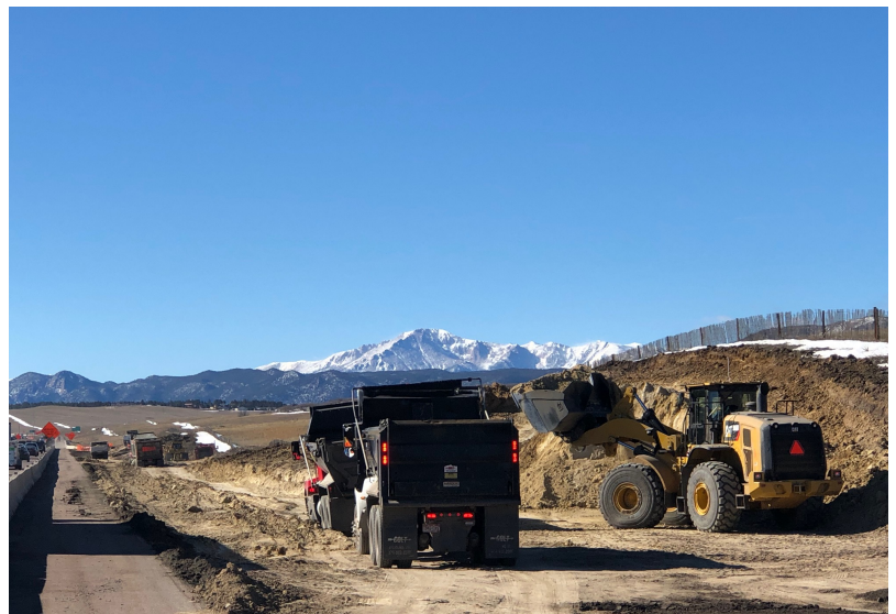
Crews perform excavation measures in the southern section of the project
