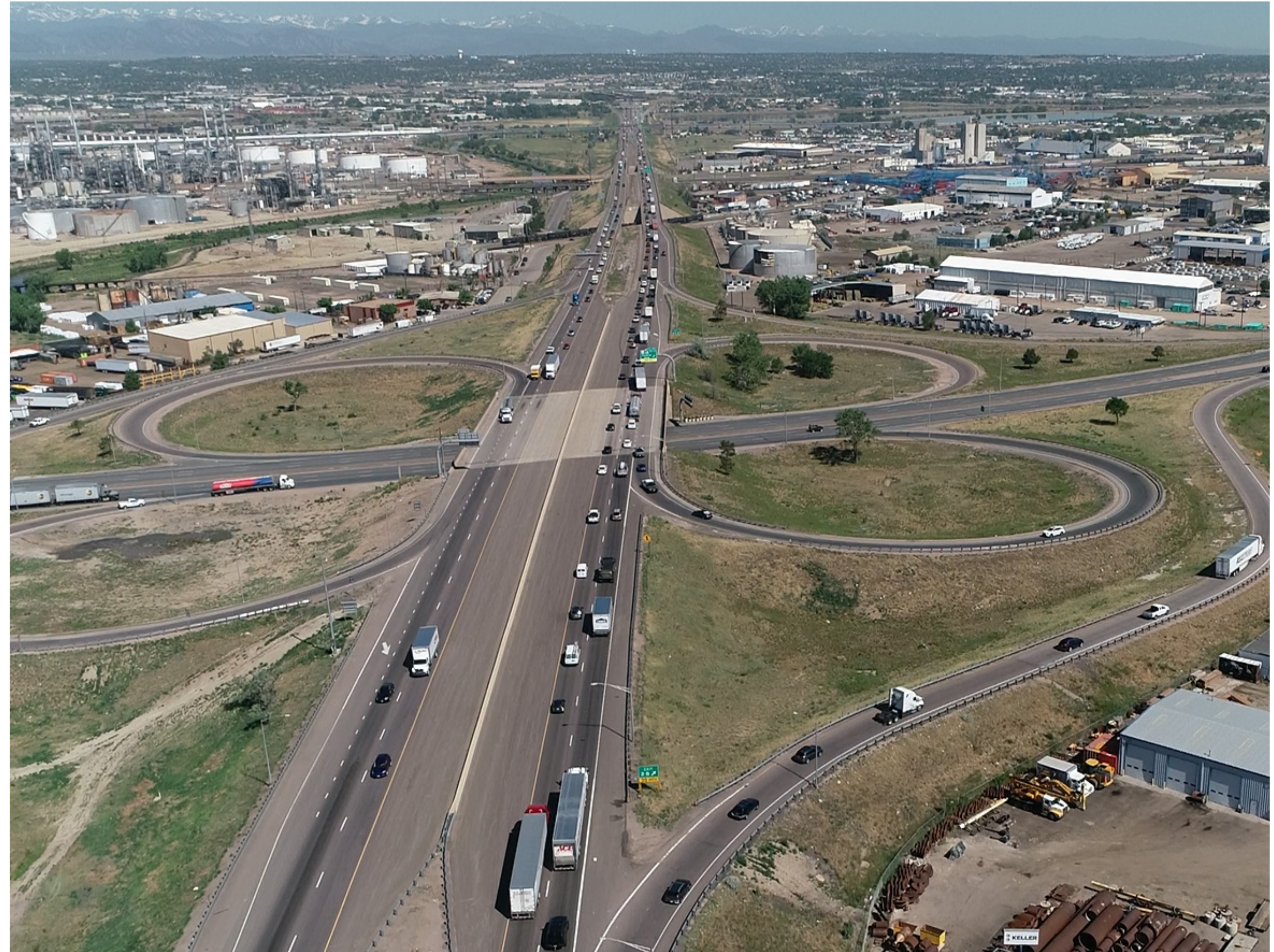
I-270 looking west from Vasquez Boulevard interchange
