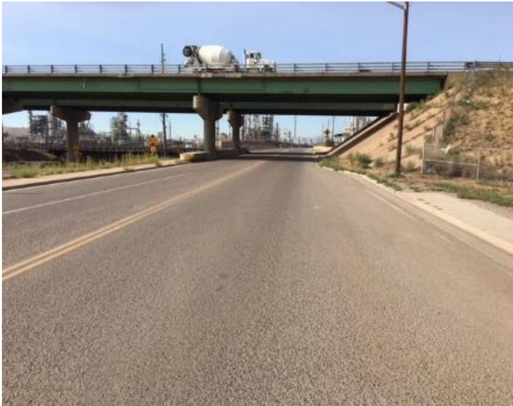
Figure 15. Brighton Boulevard Crossing Under I-270, Looking South
