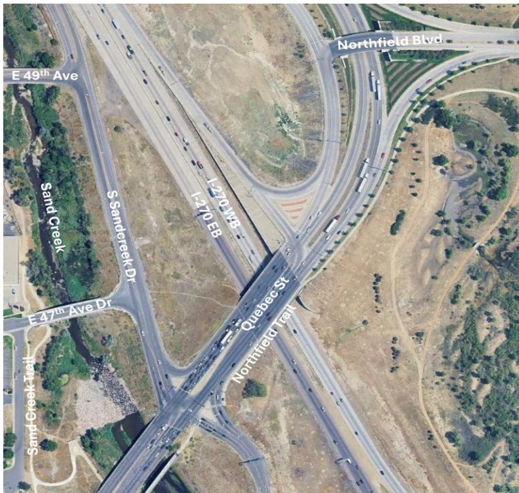
Figure 23. Quebec Street Crossing over I-270, Looking North
