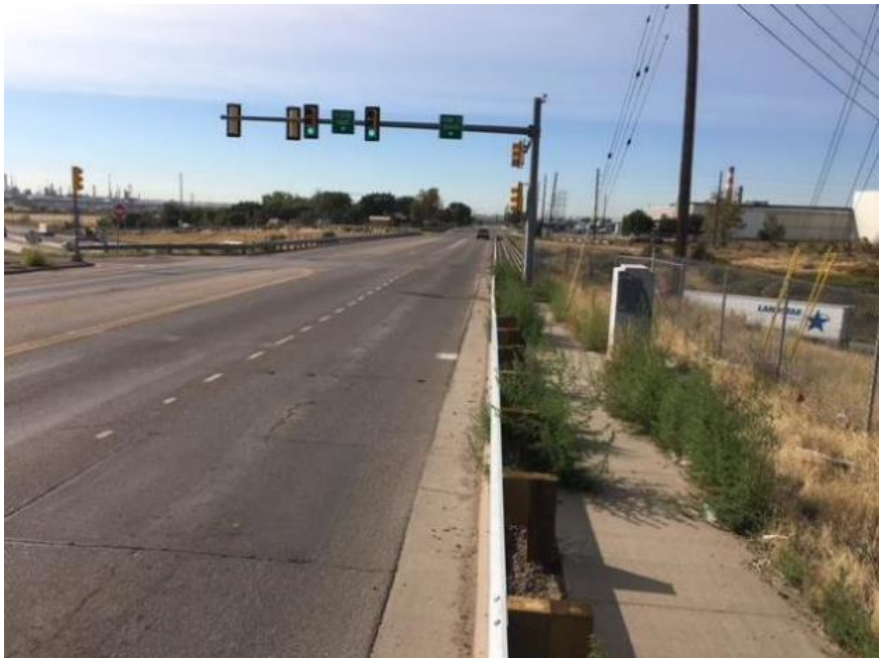
Figure 12. York Street at I-270, Looking Southbound
