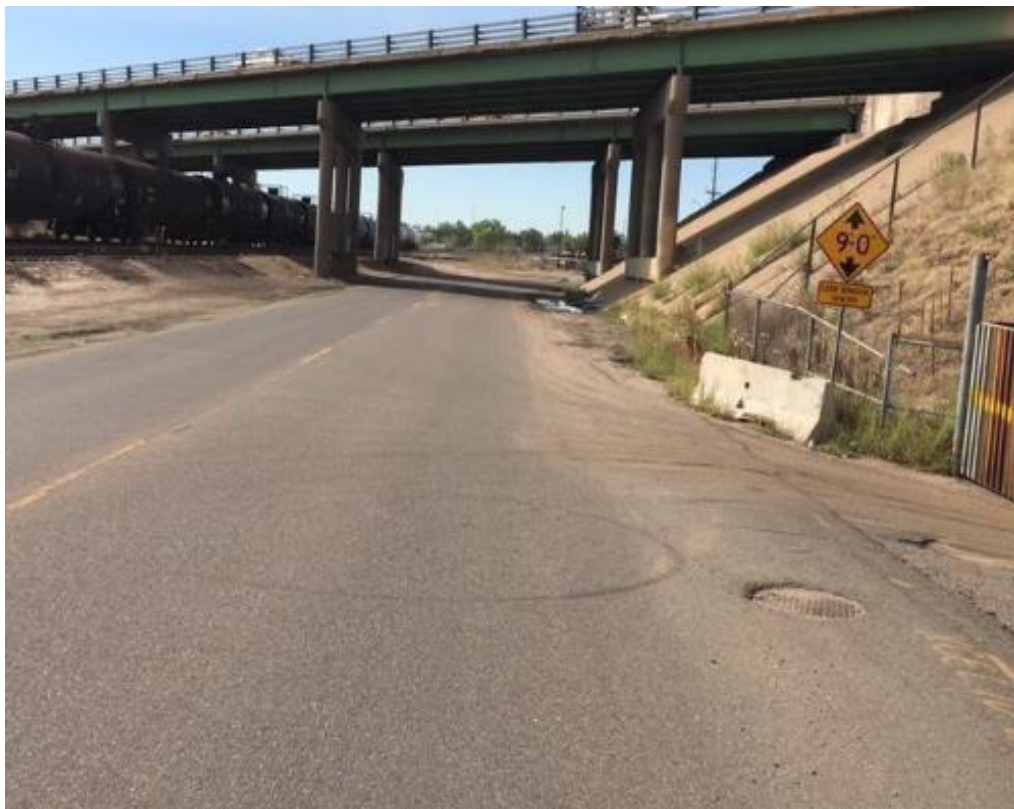
Figure 18. East 60th Avenue Crossing Under I-270, Looking South
