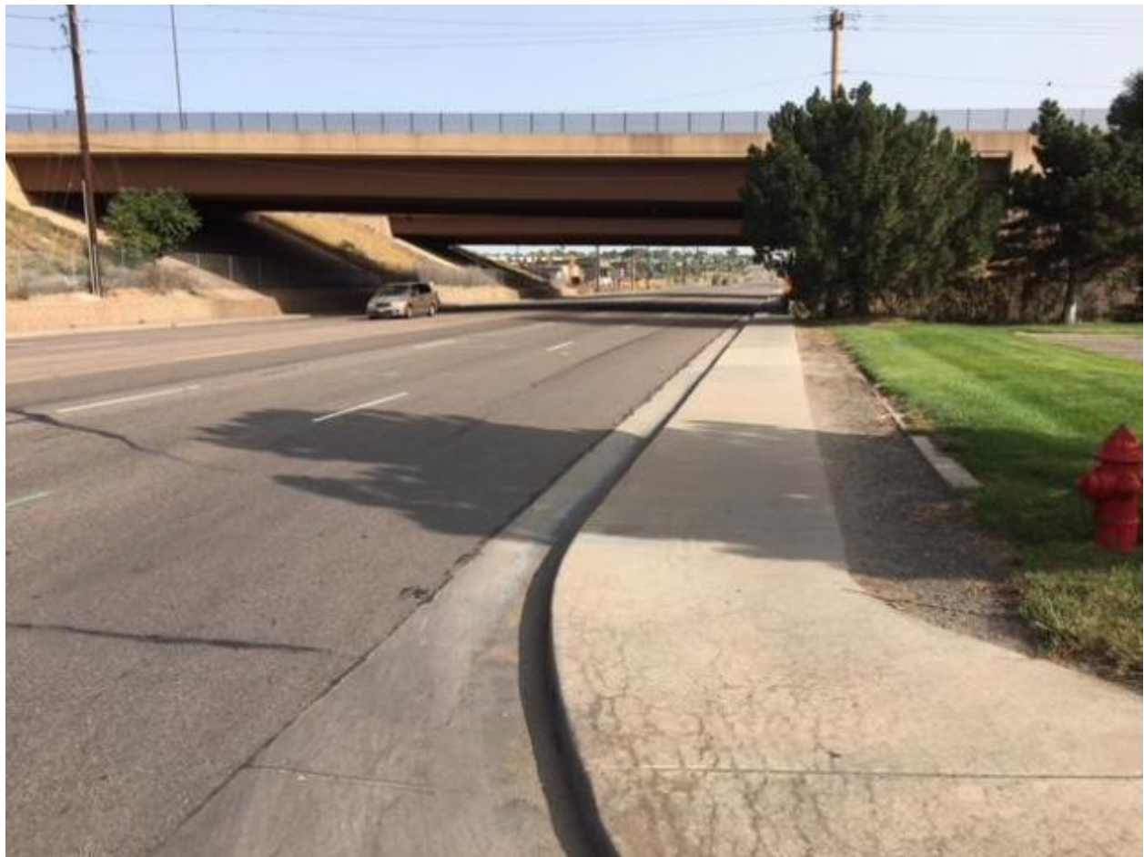
Figure 10. Washington Street at I-270 Looking Northbound
