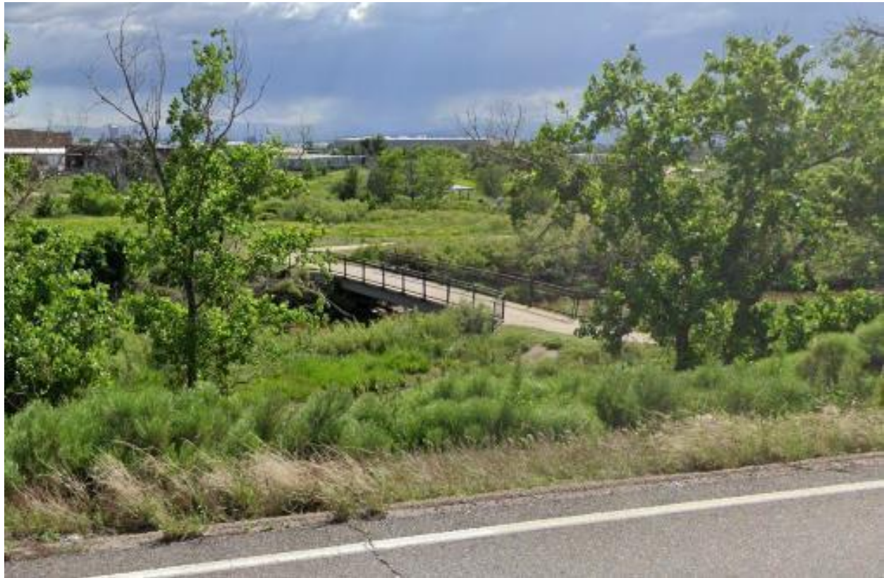
Figure 13. Connection of Wetland Park Loop Trail to Sand Creek Trail near Pedestrian Bridge
