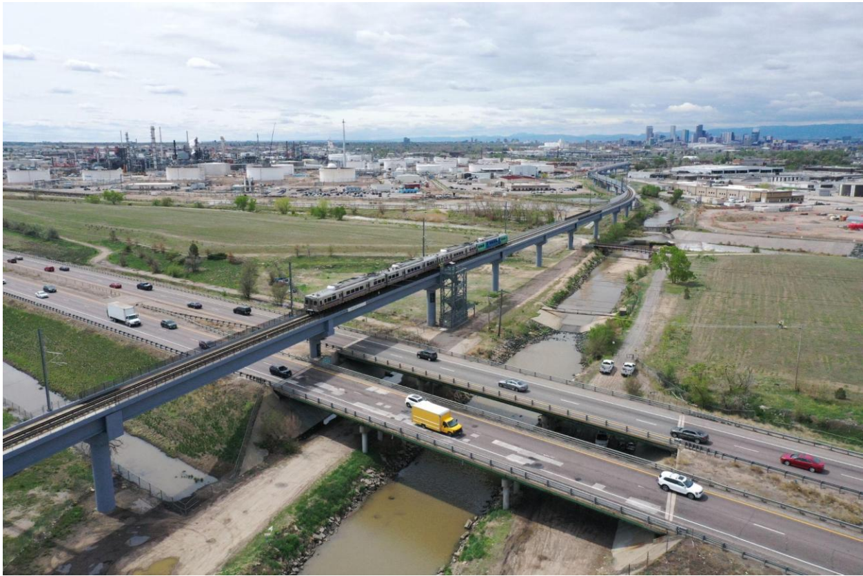
I-270 crossing over the Burlington Ditch and Sand Creek Regional Greenway trail. The RTD N Line crosses over I-270 and vacant and industrial development surrounds the corridor, facing south.
