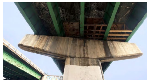
Deteriorating bridge conditions on I-270 over Brighton Boulevard
