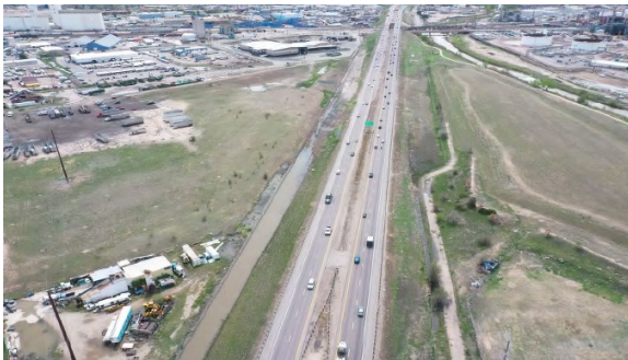
I-270 looking eastbound near Burlington Ditch
