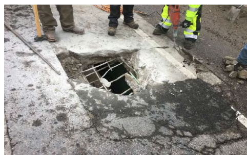
Bridge deck failure on I-270 over the Burlington Canal
