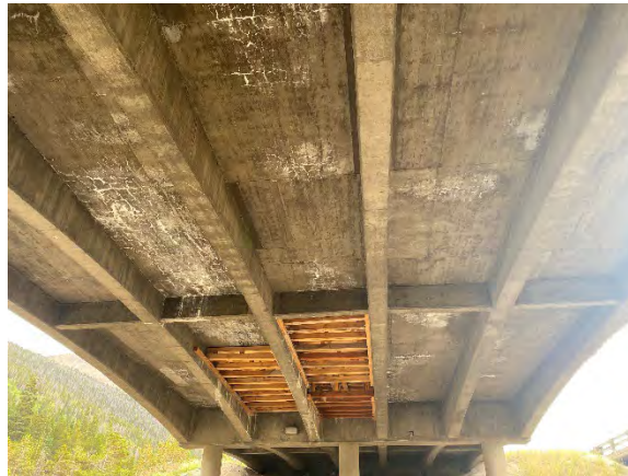
Figure 43. General view of the underside of the deck in Span 2
