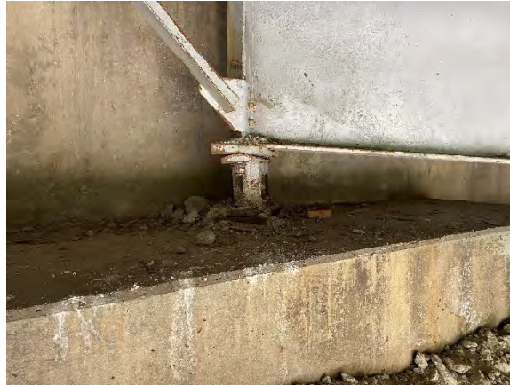
Figure 26. Typical condition of movable bearings, Abutment 1 Girder B
