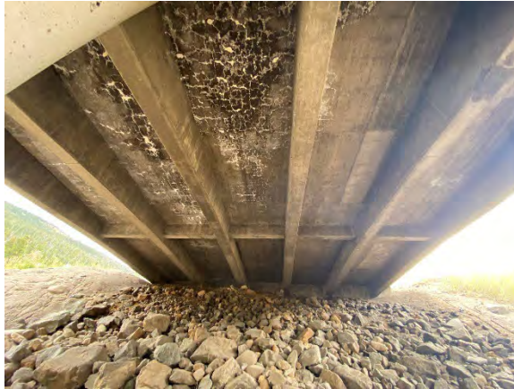
Figure 44. General view of the underside of the deck in Span 3
