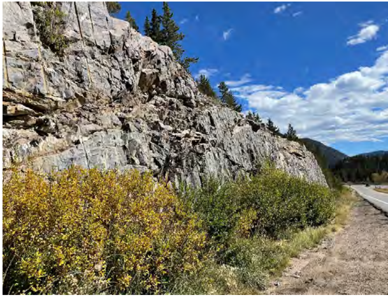
Figure 71. Bakerville exit presplit rockcut
