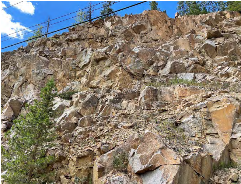
Figure 72. US 6 cushion blast type rockcut
