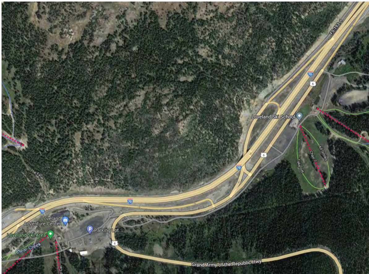
Figure 3. Aerial view of I-70 at the US 6 Interchange and Loveland Ski area
