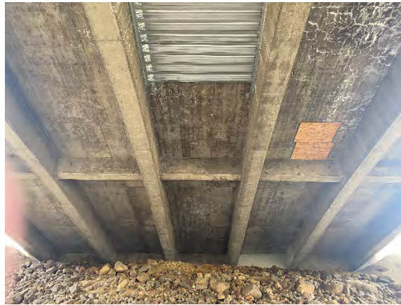
Figure 42. General view of the underside of the deck in Span 1
