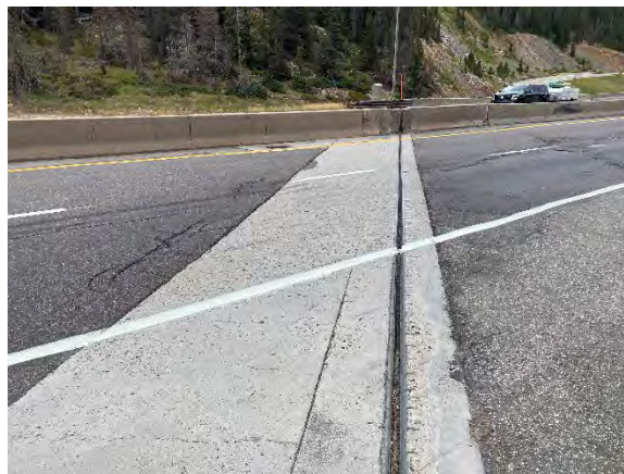
Figure 21. Expansion joint at Abutment 1
