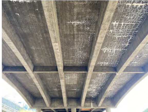
Figure 32. General view of the underside of the deck in Span 2
