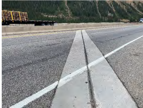
Figure 9. Expansion joint at Pier 2
