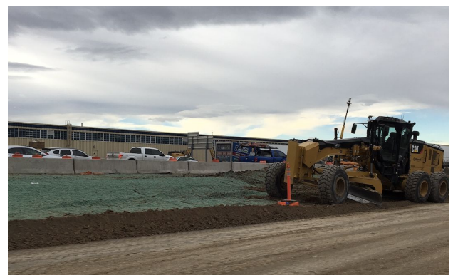
Covered dirt along Stapleton North Drive, December 2019
