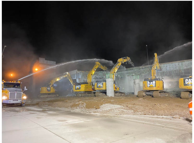
Water trucks during the Brighton Boulevard bridge demolition, February 2020
