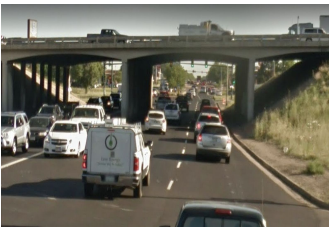
Peoria Street before construction in 2017.
