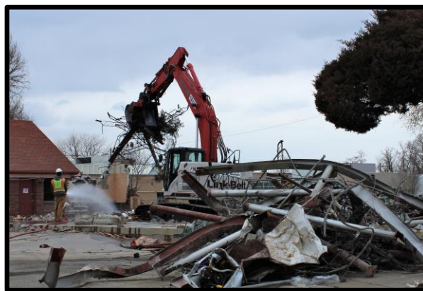
Construction crews spray water at the Colonial Manor Motel demolition site
