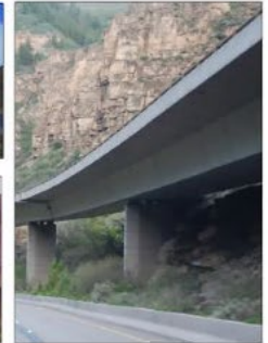
B | Deep overhangs and shadow lines add visual depth and give the bridge superstructure a thin appearance.
