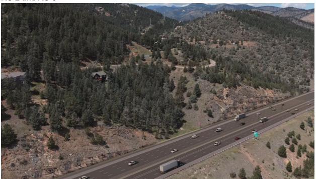
The Project Team described the options for the rock cut sections RC-2 and RC-3. These include a direct vertical cut with stabilization (a wall) or a rock cut that would lay back at a 30 degree slope to avoid risk of failure. The engineers recommended the vertical rock cut with a structural support wall at the base to ensure stability. The rock cut that would lay back 30 degrees would remove slope vegetation and potentially destabilize the road above that slope.
