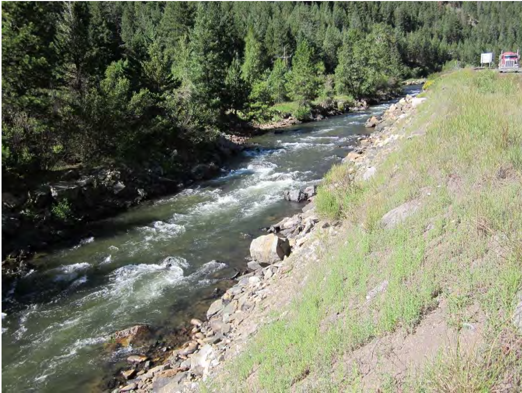
Photo Point 20: Facing upstream, this reach of Clear Creek is confined by a steep embankment to I-70 and a rip rap-stabilized right bank.
