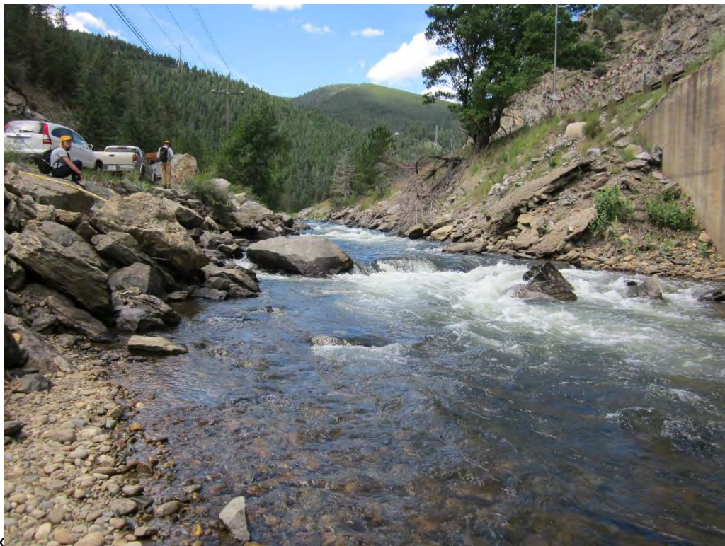
Photo Point 26: Near Hwy 6/I-70 merge facing upstream, this reach is channelized with rip rap and concrete walls.
