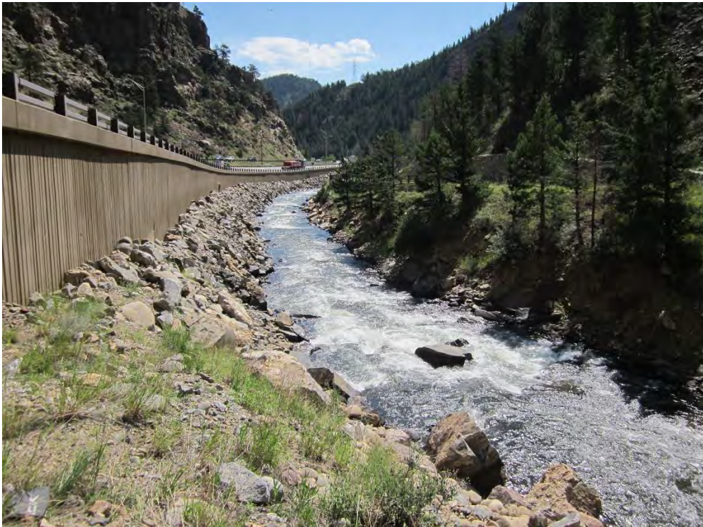
Photo Point 4: Facing downstream on a reach of Clear Creek. The channel is confined between rip rap along I-70 on the left bank, and a rip rap-stabilized bank on the right.
