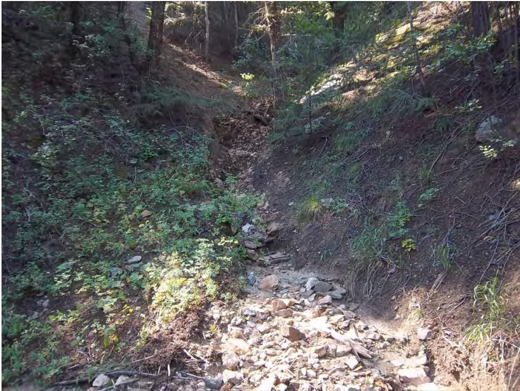
Photo Point 34: Drainage OW2, an intermittent or ephemeral tributary to Clear Creek. Facing upstream from the trail, a culvert carries it to wetland WL24 from this point.
