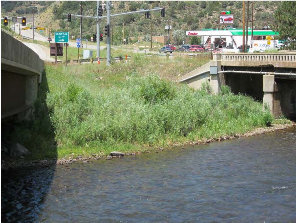
Photo Point 13: Wetland WL14 is mostly narrow-leaf willow and Baltic rush, confined to the bank between bridges. Facing west from the opposite bank.
