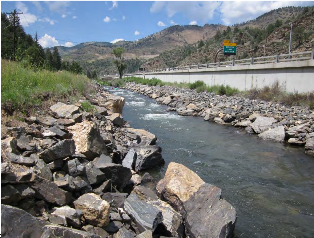
Photo Point 17: Facing upstream, this reach of Clear Creek is confined by rip rap on both banks, I-70 on the left bank and the trail on the right bank.
