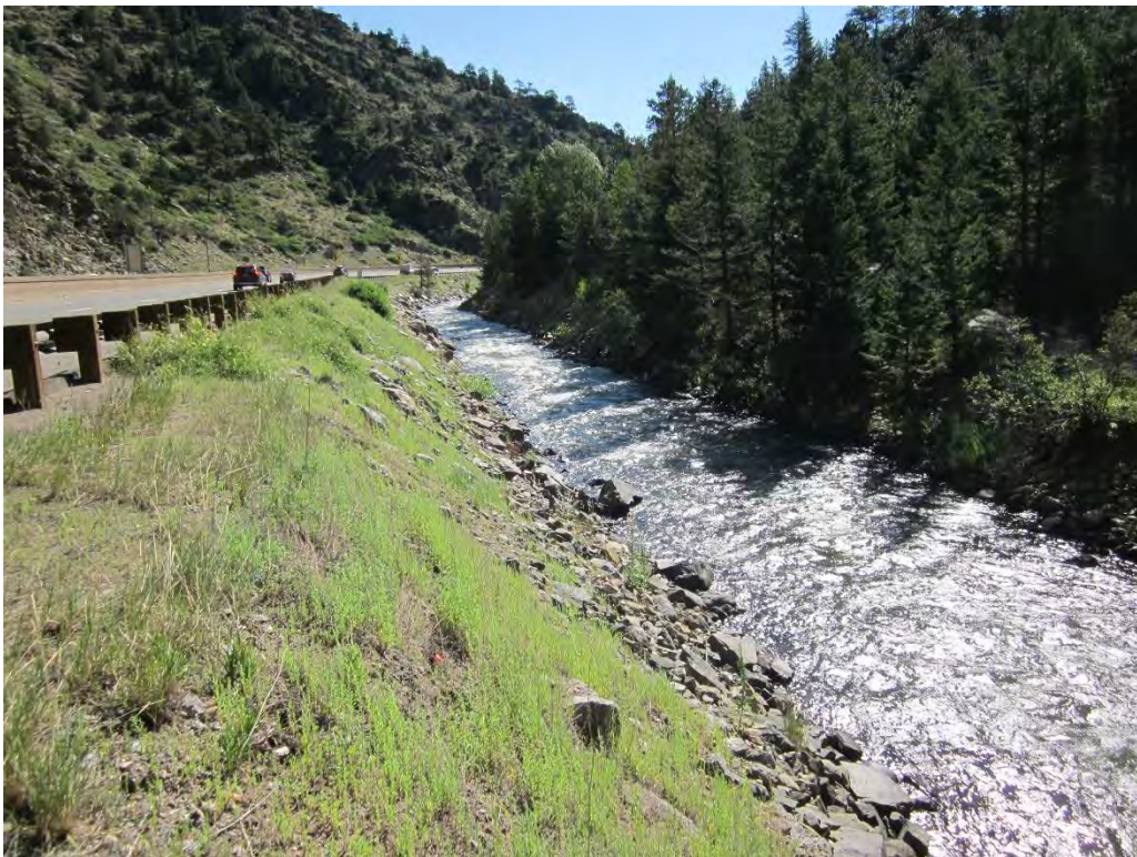
Photo Point 20: Facing downstream, channelization has prevented floodplain and wetland development through this reach.
