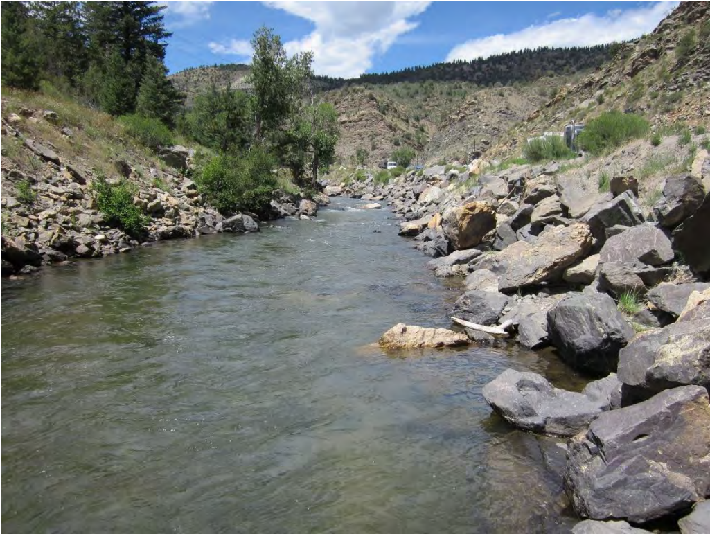
Photo Point 29: Rip rap stabilization continues downstream from Photo Point 28, facing upstream.
