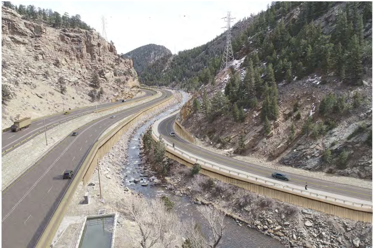
6 7 These alignment shifts would result in substantial rock cuts on both the north and south sides of the 8 canyon (see Exhibit 38). On the north side, rock cuts up to 160 feet high would be required next to the
