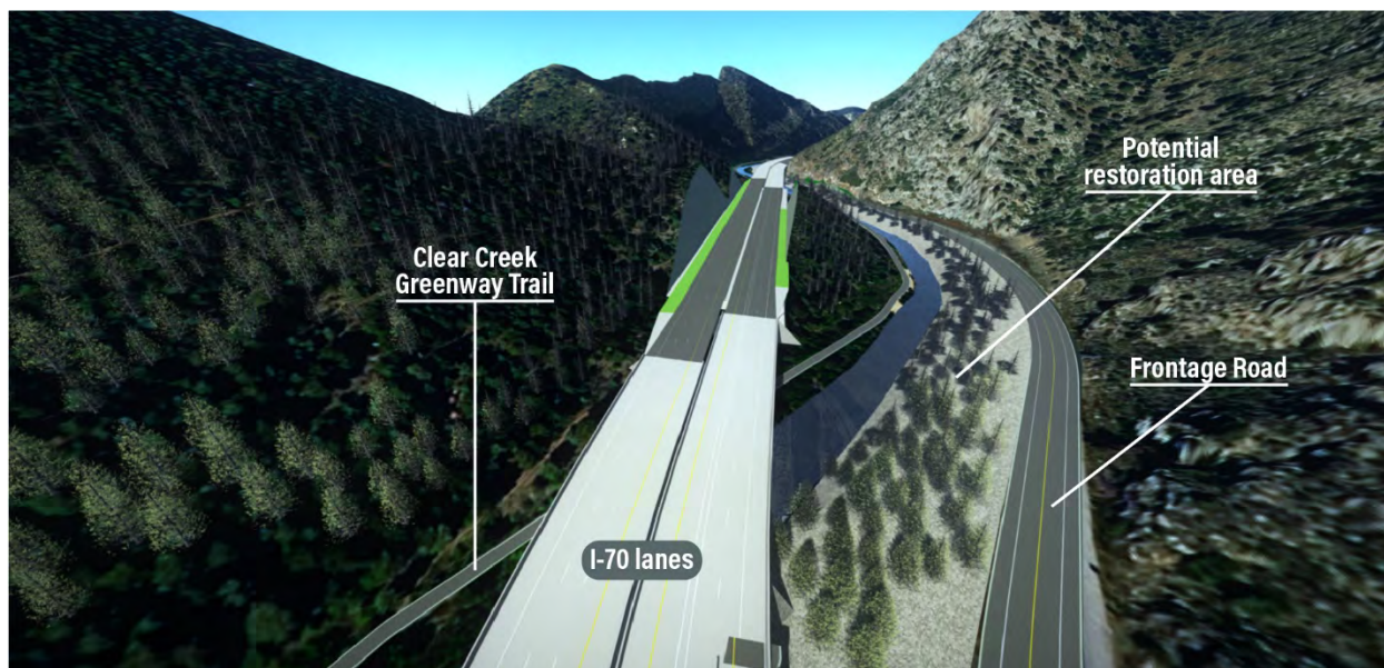
1 Exhibit 33. Canyon Viaduct Alternative - Viaduct Structure, Bench Cut in Hillside, and Clear Creek 2 Restoration Area Between US 6 and Hidden Valley/Central City Interchanges; Looking West
