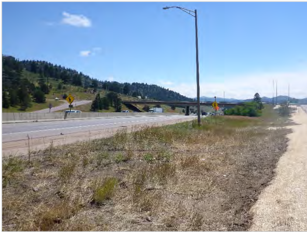
Photo 7. Looking east from the west side of the Hyland Hills/Floyd Hill interchange bridge in the I-70 highway right of way (ROW) near MP 246.5 during the summer of 2017.
