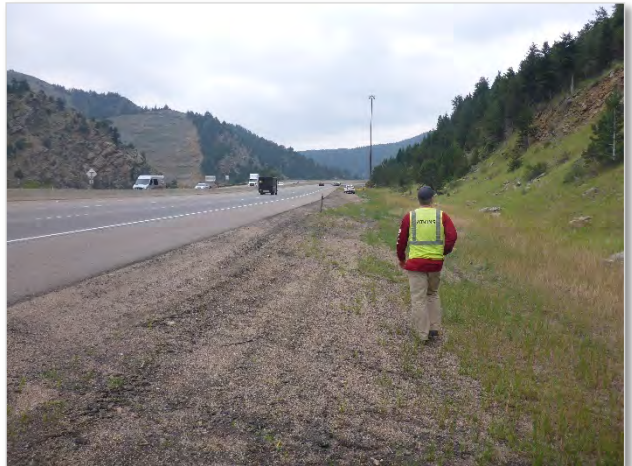
Photo 12. Looking east from the bottom of Floyd Hill at the vegetation and topography leading to the top of Floyd Hill near MP 245 during the summer of 2017.
