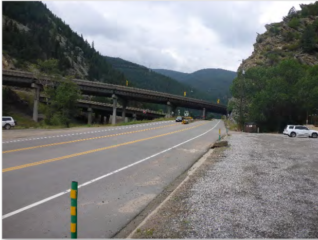
Photo 17. Photo looking east at the I-70/US 6 interchange, with Clear Creek on the left near MP 244.5 during the summer of 2017.
