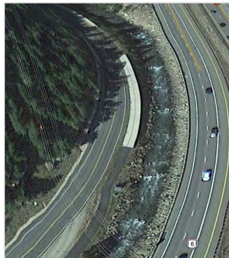
Photo 7. Clear Creek Realignment Area
