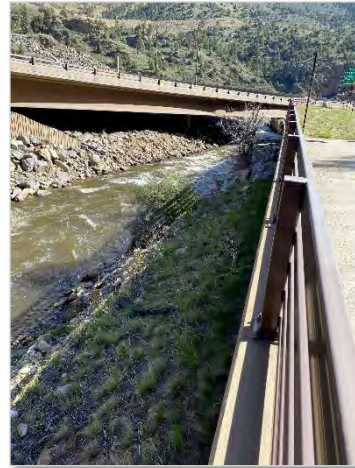
Photo 24. Picture looking east along East Idaho Springs Road west of the Hidden Valley/Central City interchange near MP 242.7 in May of 2020. Shows the narrow riparian corridor and the steep riprapped banks.
