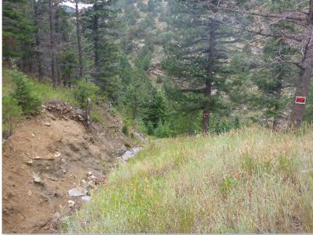
Photo 13. Example of slopes and drop-off of several gulches (Sawmill and Johnson) that intersect I-70 in the Study Area near MP 245 during the Summer of 2018.
