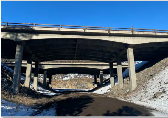
Photo 6. Existing bridge over Soda Creek Road MP 249
