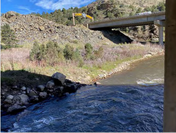
Photo 25. Picture looking east at the Central City Parkway Bridge over Clear Creek near MP 242.8 north of I-70. Example of the narrow riparian corridor adjacent to Clear Creek.
