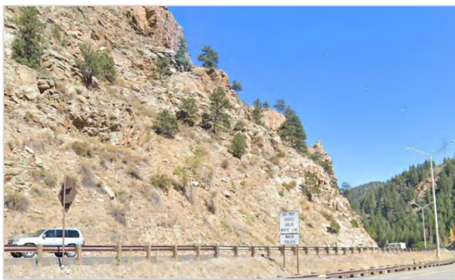
Photo 3. Rock Cut Area, North Side of I-70
