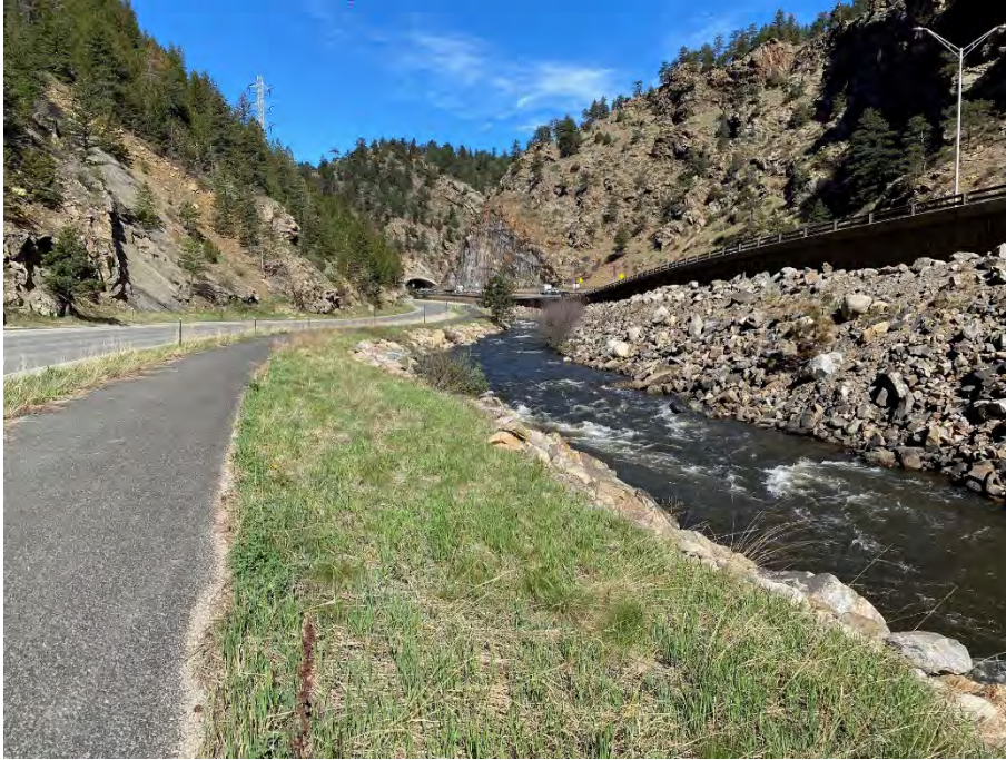
Photo 5. Clear Creek Realignment Area
