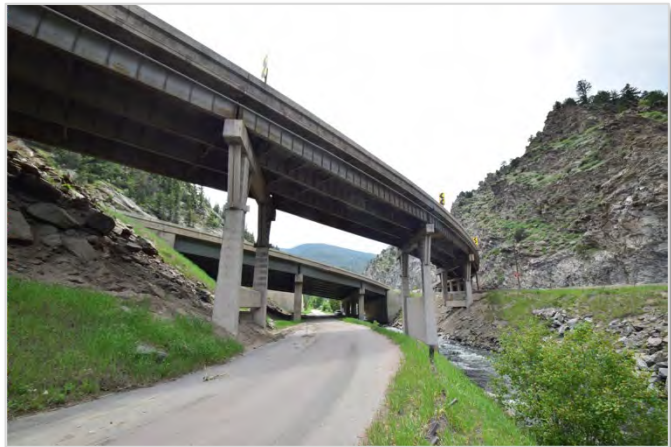
Photo 2. Existing bridges over Clear Creek and the recreation trail at MP 244.2
