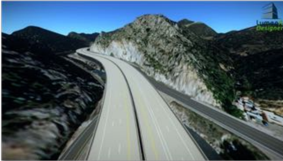
East Portal – Looking West (Figure 4)
