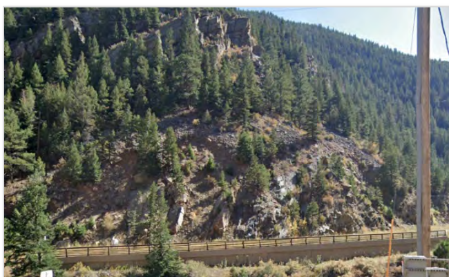
Photo 4. Rock Cut Area, South Side of I-70
