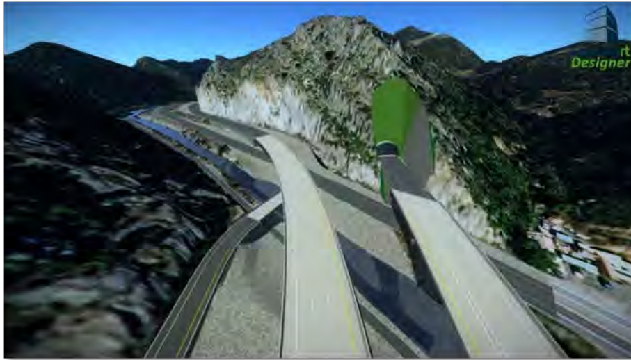
East Portal – Looking West (Figure 1)
