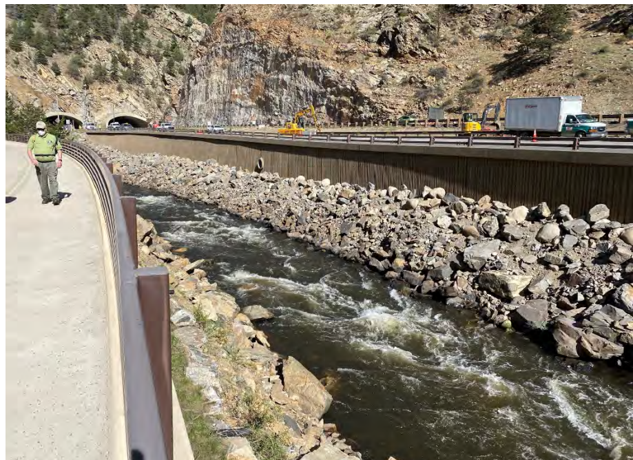
Photo 6. Clear Creek Realignment Area
