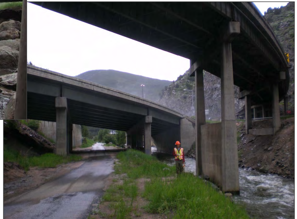
Clear Creek/ US 6 Interchange
