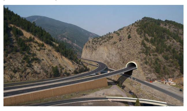
At I-70 and US 6, the project will maintain the existing WB I-70 exit-ramp and add an EB I-70 on-ramp. US 6 will be extended to the west providing additional access to and from I-70 at the Hidden Valley interchange with Central City Parkway and will connect with CR 314. WB will be placed in tunnel. Greenway trail will be improved from US 6 to VMT.
