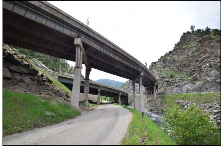
Existing I-70 bridges spanning the bike path, Clear Creek & the I-70 westbound on-ramp.
