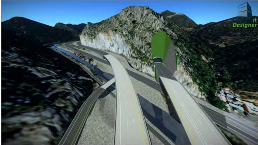
East Portal – Looking West (Figure 1)
