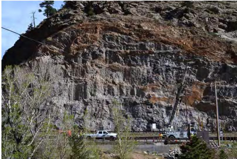
Rock excavations and rock cuts in the I-70 Mountain Corridor need to be carefully designed, and rockfall mitigation measures need to be included to avoid long-term maintenance and safety issues. The design and review of rock cuts will be coordinated with the CMGC to minimize potential hazards.
