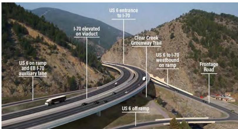
As illustrated in [Exhibit 3-8](#), realigning the roadway on the south side of the canyon would avoid existing tight curves around the two hills between the US 6 interchange and the Hidden Valley/Central City interchange (west of the view in [Exhibit 3-6](#)). Elevating I-70 would provide more space in the canyon for the new frontage road (allowing it to be constructed generally within the existing I-70 pavement), creek, and wildlife movement and would create opportunities for
