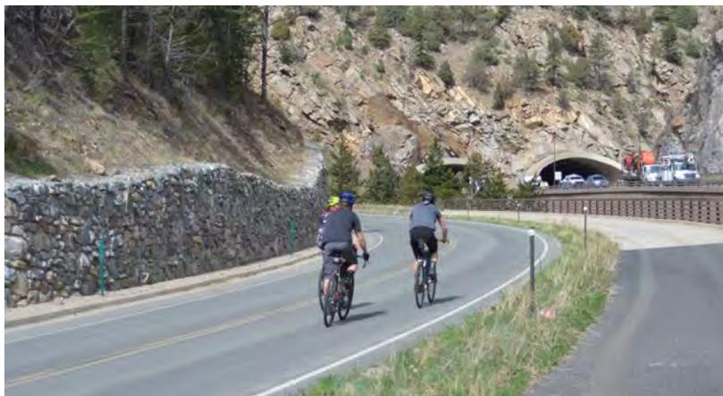
While mitigation measures both in design and construction would be similar to those described for the Canyon Viaduct Alternative, the scale of rock cuts and proximity to I-70 travel lanes significantly complicate the design, construction, and maintenance of the Tunnel Alternative. Additionally, hauling and disposing of excavated materials would be more complicated and time consuming under the Tunnel Alternative compared to the Canyon Viaduct Alternative.
