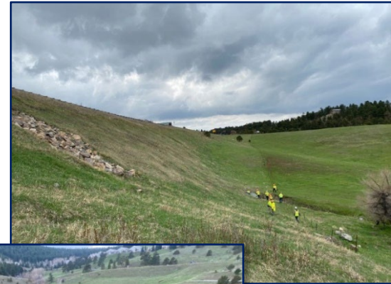
View below I-70, looking east at MP 254.4
