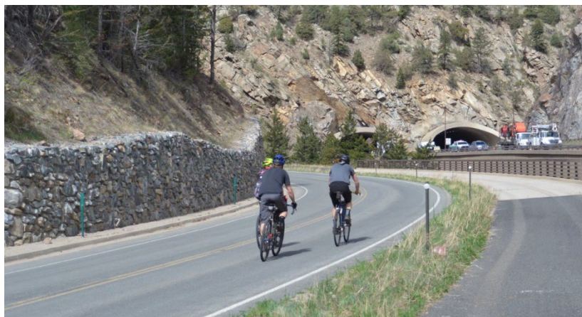
Figure 4-2 Existing Retaining Walls along CR 314 that will be Replaced after New Rock Cuts to the South
