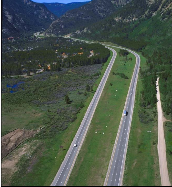
Tenmile Canyon, view southwest
