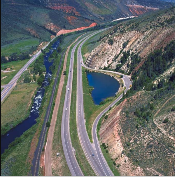
Wilmor Lake, view west
