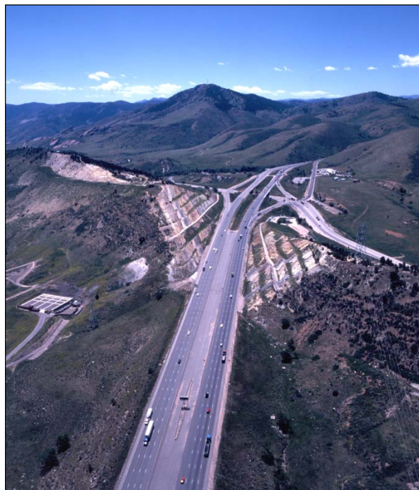
The I-70 highway cut through Hogback Ridge, view west
