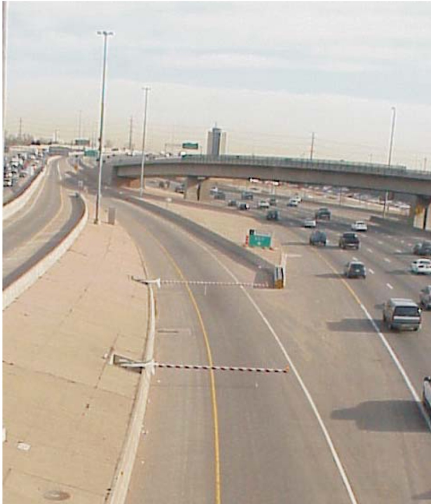
Urban example: Reversible Lanes on I-25 in Denver with gates to prevent entry during reverse direction operation.
