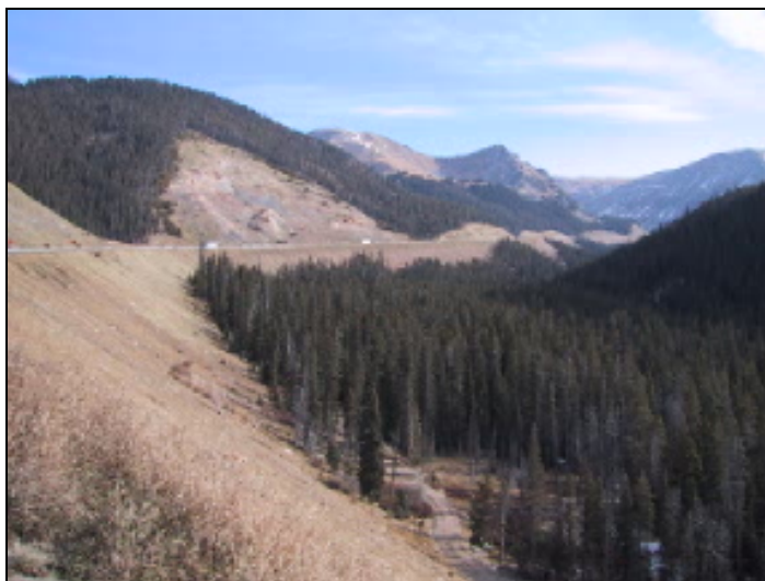
Figure 11. Poorly Vegetated Cut-and-Fill Slopes East of the Eisenhower-Johnson Memorial Tunnels
