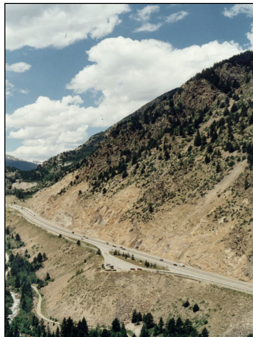
Figure 12. Rockfall Chutes along the Georgetown Incline
